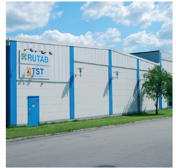
Warehouse - and production facility in Nässjö, Sweden
